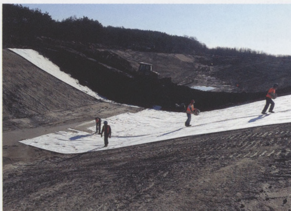
L-R: The pond lining being constructed. Tunnel construction under Leslie Street which spanned 166 feet to connect the east and west sides of the course.
