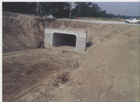
L-R: The pond lining being constructed. Tunnel construction under Leslie Street which spanned 166 feet to connect the east and west sides of the course.
