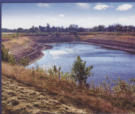
Piper's Heath reservoir was put to the test last summer with only 4,000,000 gallons to spare. (Credit: Cam Shaw)
