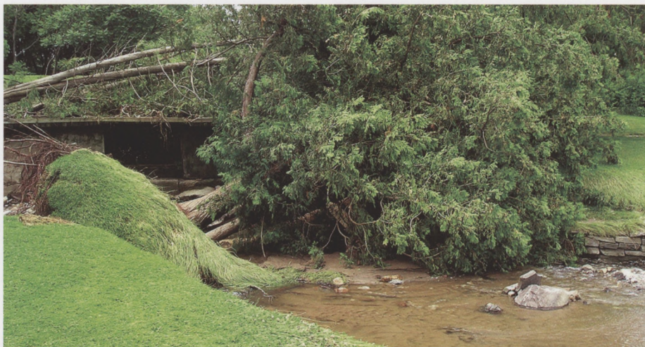
Flood damage in creek by the 12th hole, photo courtesy of Kelly Drum.
