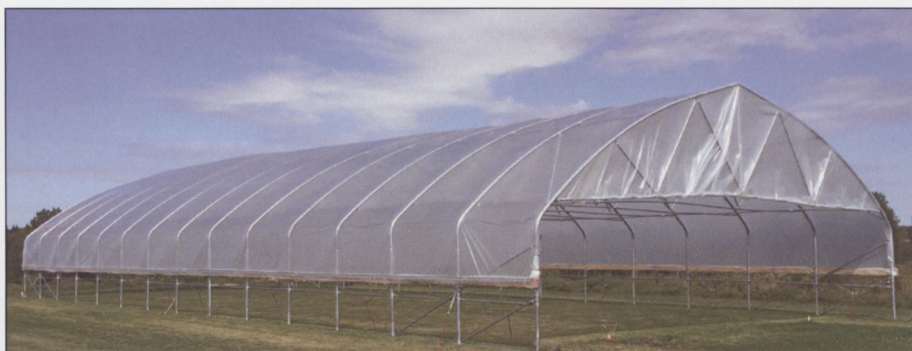
The finished rain out device seen here with the plastic covering installed to inhibit precipitation and maximize light penetration.
