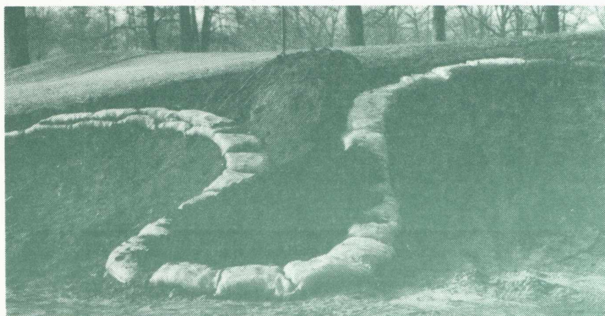
But soil-filled burlap bags work better.
