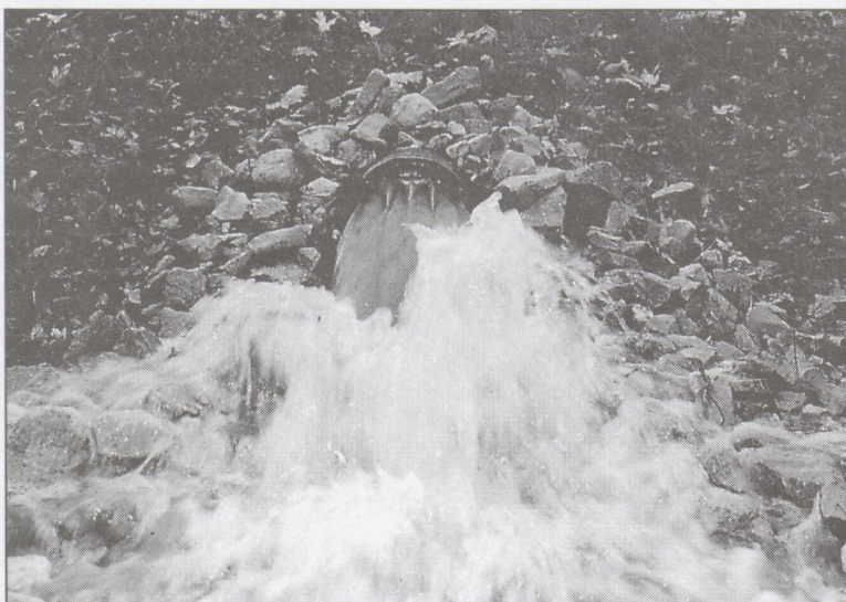
GO WITH THE FLOW! TURF DRAIN INC. DRAINAGE INSTALLATION
