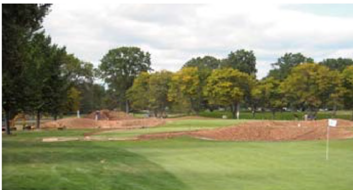
(Green complex during the shaping process - notice temporary green within fairway)
