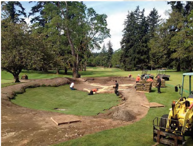
Photos (Above and below) courtesy of Joel Kachmarek, GCS - Sod under bunker - to be sprayed with Round-Up then add bunker sand.
