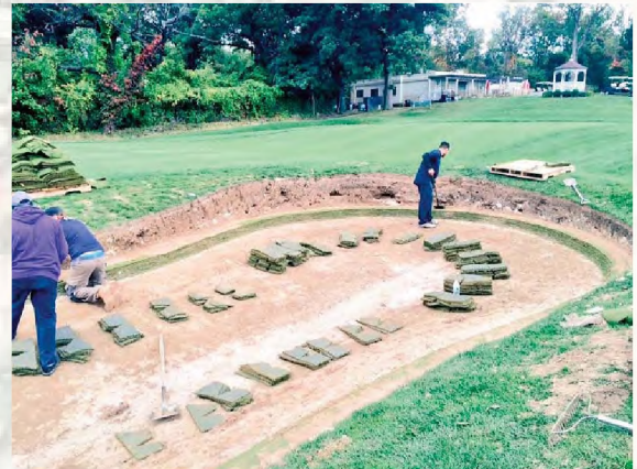
Above & Below: Mosholu GC in the Bronx - 9th Hole installing Ecobunker to create revetted bunker
