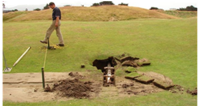
A failed join across the 3rd fairway mainline which requires a $600 coupler and many hours of labour to repair. With little to no isolation, this breakage "took down" the entire system.
