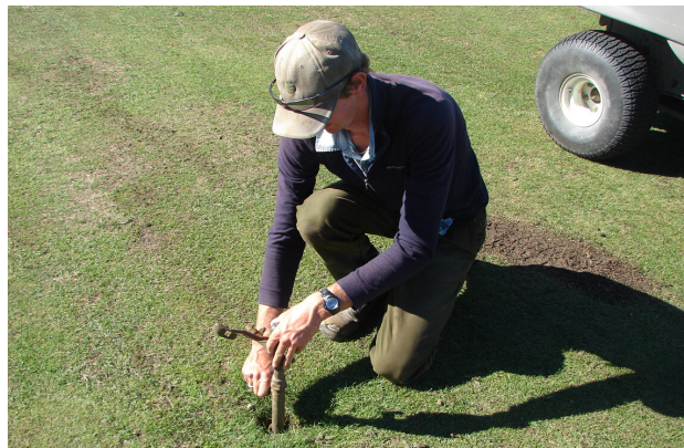
The system required a large amount of manual control and labour with all the fairways being irrigated by above ground sprinklers which are shifted cyclically in season (daily).
