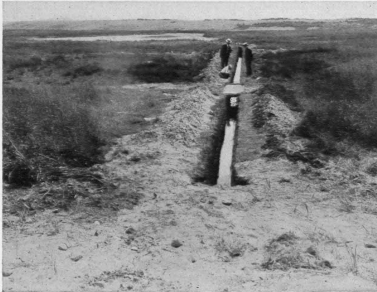
Swampy areas too extensive to permit filling in may be effectively rid of mosquitoes by means of properly constructed ditches. The main ditch for the area here shown is two miles long, draining at each end into a rocky beach.
