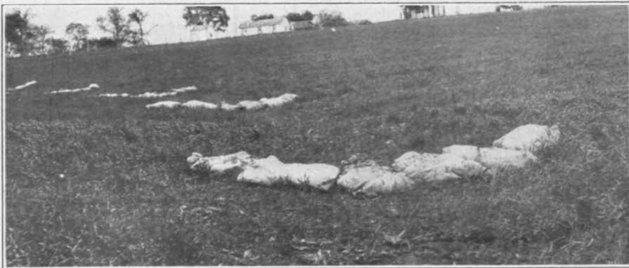
The formation of gullies can be checked by sodded dams constructed by placing burlap bags filled with sod in any depression which serves as a channel for conveying the runoff from a field terrace on a higher slope. This is a wide depression and thus required a great number of bags
