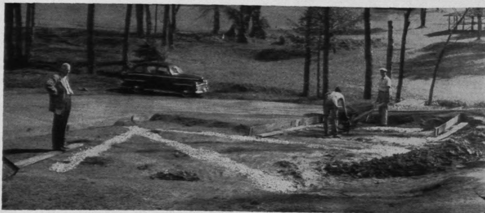
Alex G. McKay, the author, inspects the sub-surface drainage system while workmen haul topsoil. Mr. McKay uses the herringbone drainage pattern and believes whole-heartedly in sub-surface drainage for best results with bentgrass greens in the South.
