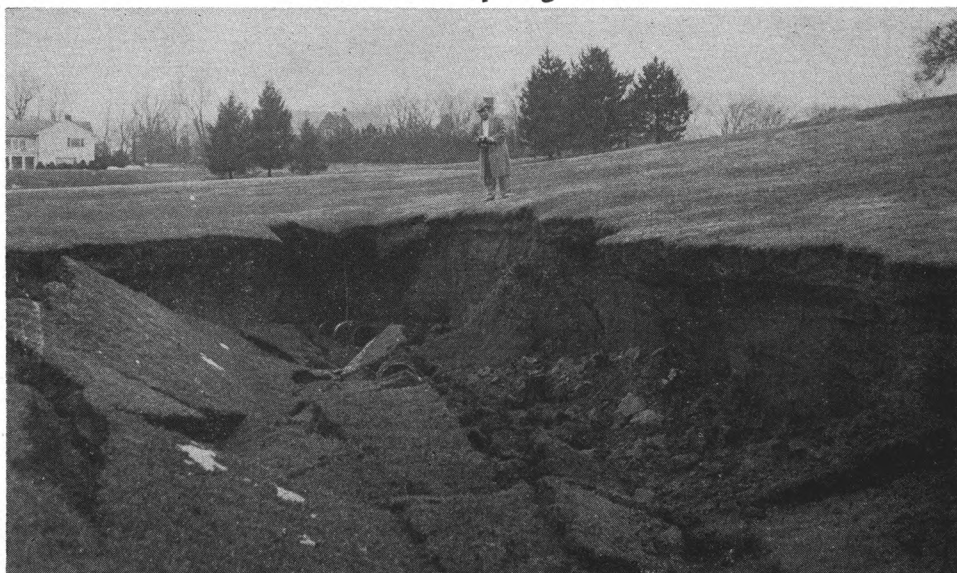
This is what the spring rains did to the eleventh fairway of Woolfert's Roost Country Club, Albany, N. Y. A heavy three-inch rainfall overburdened a storm sewerage line causing it to break. Here, Mr. Jack Gormley, Superintendent, surveys the damage. In some areas of the fairway the soil deposit resulting from the break measured approximately two feet in depth.
