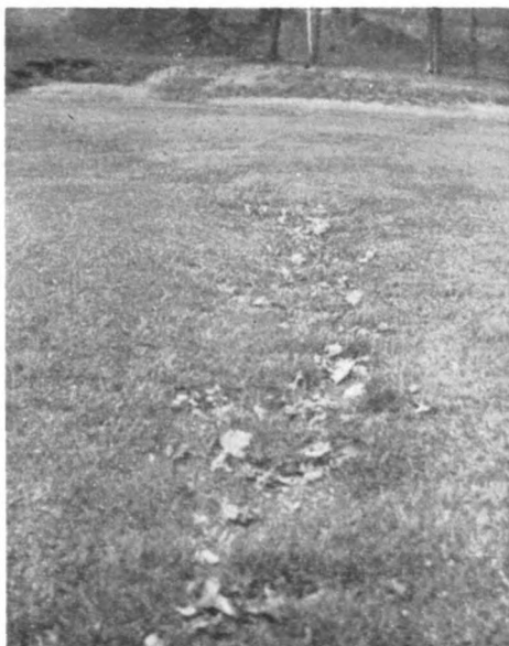
A sunken drain across the middle of a fairway at the Montclair Golf Club caused this depression to appear at the fifth hole, third nine.
