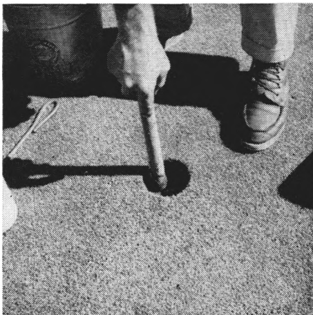
. . . and is tamped with stick.
