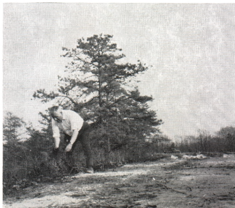
Eb Steineger raising a "blanket" of vegetation lifted from adjacent areas to cover slopes of the new tee, giving it that "natural look."
