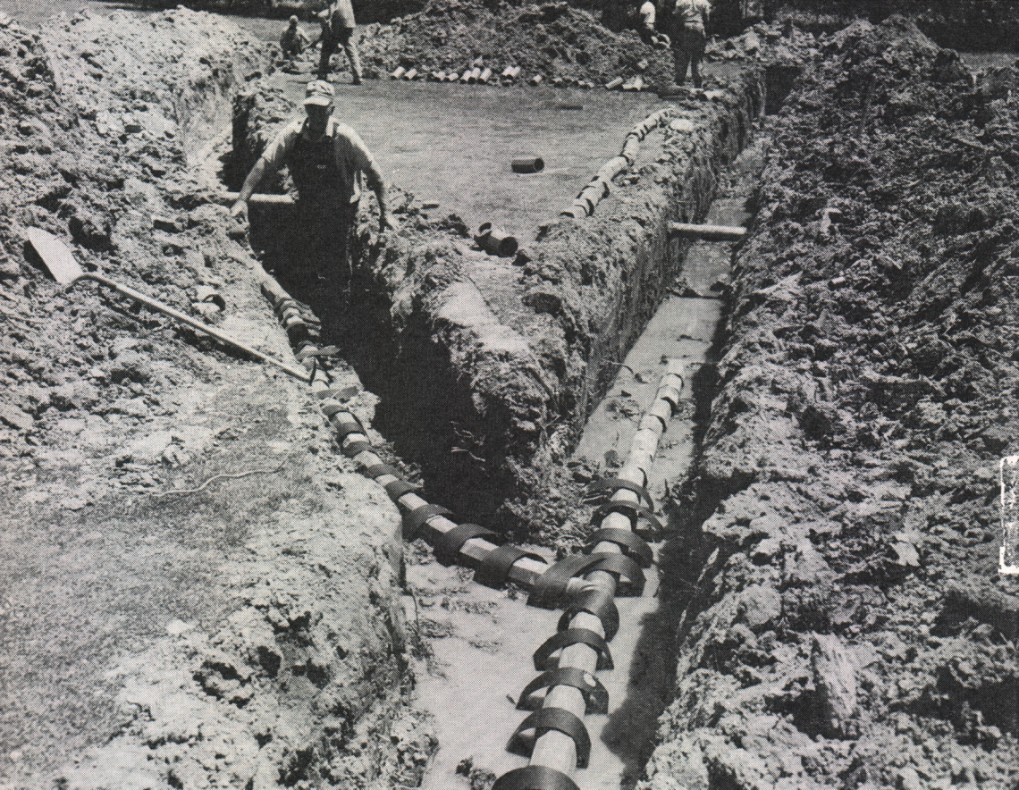
Tiles are being placed to effect rapid removal of water seeping into the trench. Note the strips of tar paper which were to be used to cover the joints, thus keeping gravel or soil from falling into the tile line. Note also the abundance of tree roots growing out from the sides of the ditch.
