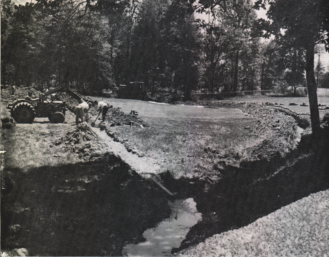
The job at Congressional is nearly complete. Tile has been installed, the gravel backfill is in place. Now a small amount of soil will be replaced and the sod laid back and tamped smooth, ready for the Open.
