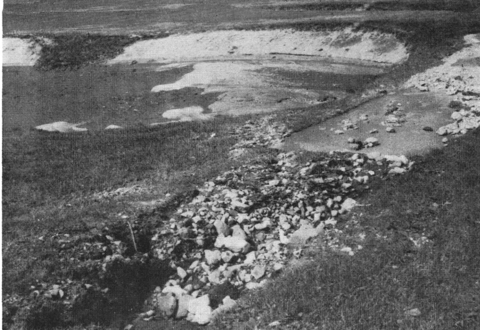
Erosion problems are accentuated at beginning of hardtop paths. Car, cart, and foot traffic wear the turf and a minor erosion problem could quickly develop into something big. Path leading away from No. 7 green at Woodbride Country Club, Woodbridge, Conn. the day after a heavy rainfall.
