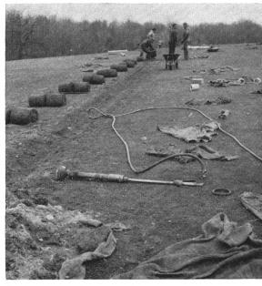
row down-the-middle arrangement of fairway sprinklers, he may observe that even with speed control for the overlapped and non-overlapped areas, the pattern of distribution is not satisfactory. The precipitation rate close to the sprinkler is far too high and the droplet size required to reach halfway across a wide fairway is much too large for satisfactory results.
