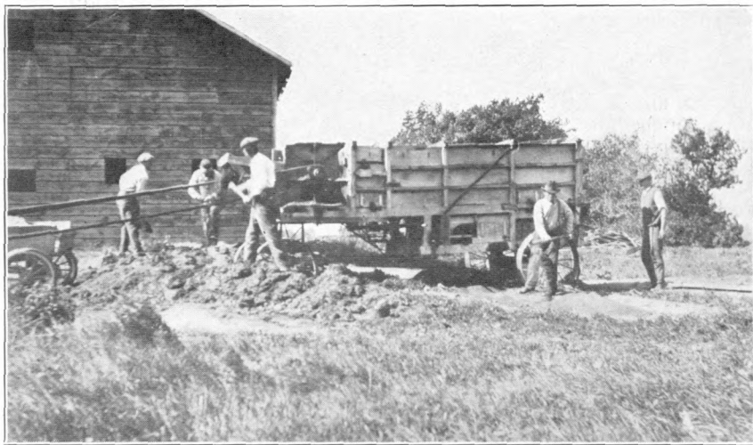
Figure 2. Mixing compost with an old threshing machine
