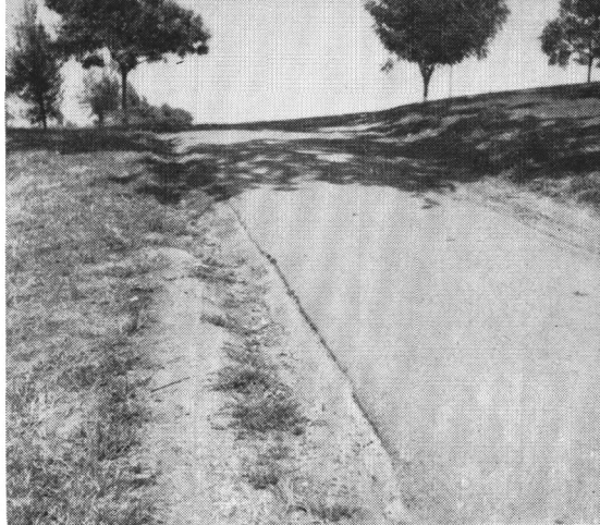
Water was encouraged to run off to the sides of this path, causing the erosion shown along the edge.
