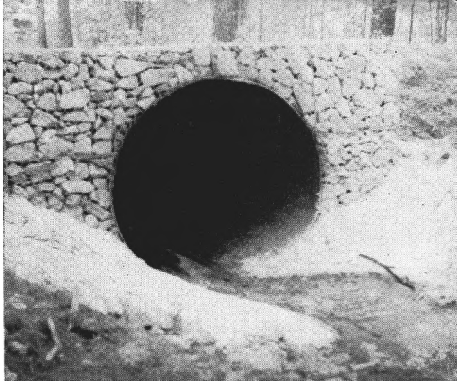
The beginning of the 640 feet of the 84" metal drain pipe laid at 2.5% grade with two reinforced concrete catch basins.
