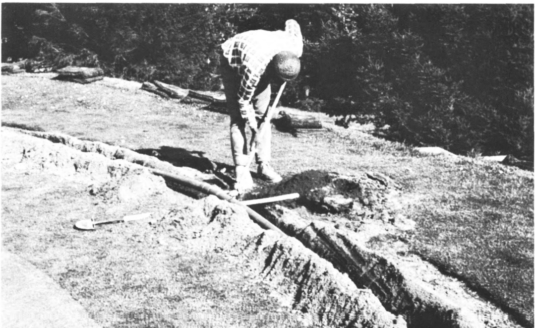
Figure IV, trenching method of laying pipe.
