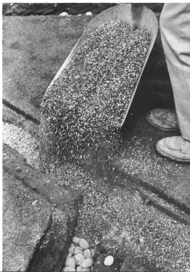
Backfilling the drain lines with graded gravel to be followed with sand. The original sod (with a sand base) will then finish the job.
