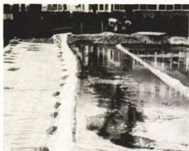
COVER PHOTO: The terrace was flooded to check for leaks in one step of building a Purr-Wick putting green.
