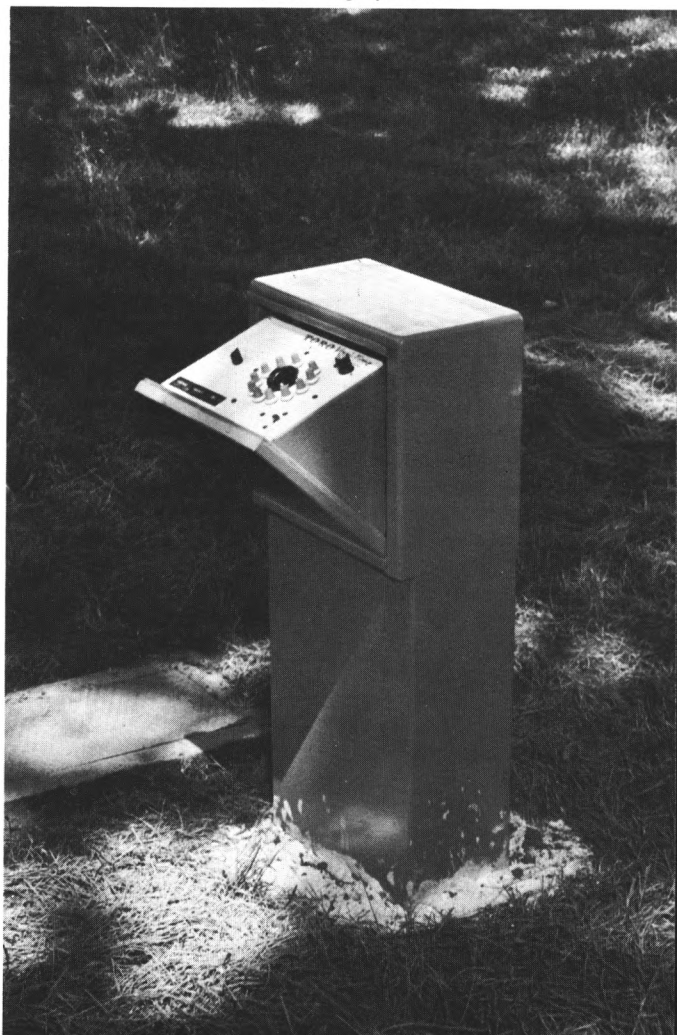
Pedestal mount controller for an underground irrigation sprinkling system.
