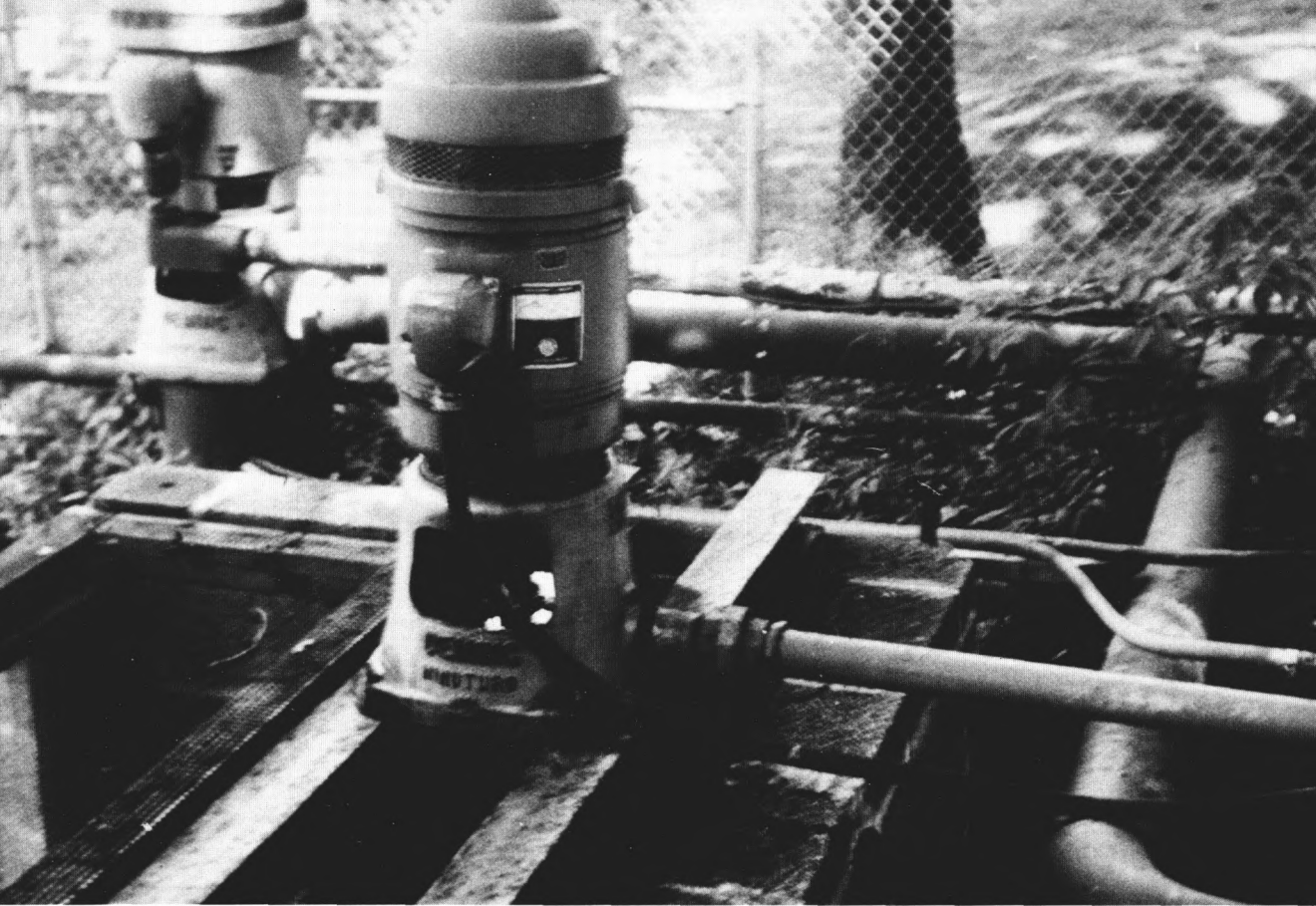
The pump used in feeding the water onto the course through kicker type sprinklers.
