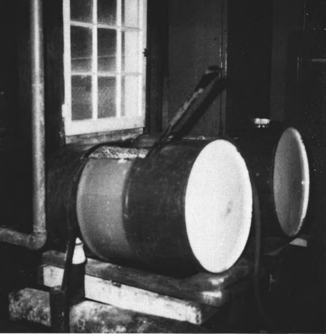
Two 50-gallon steel drums where water and fertilizer are added in the pump house.
