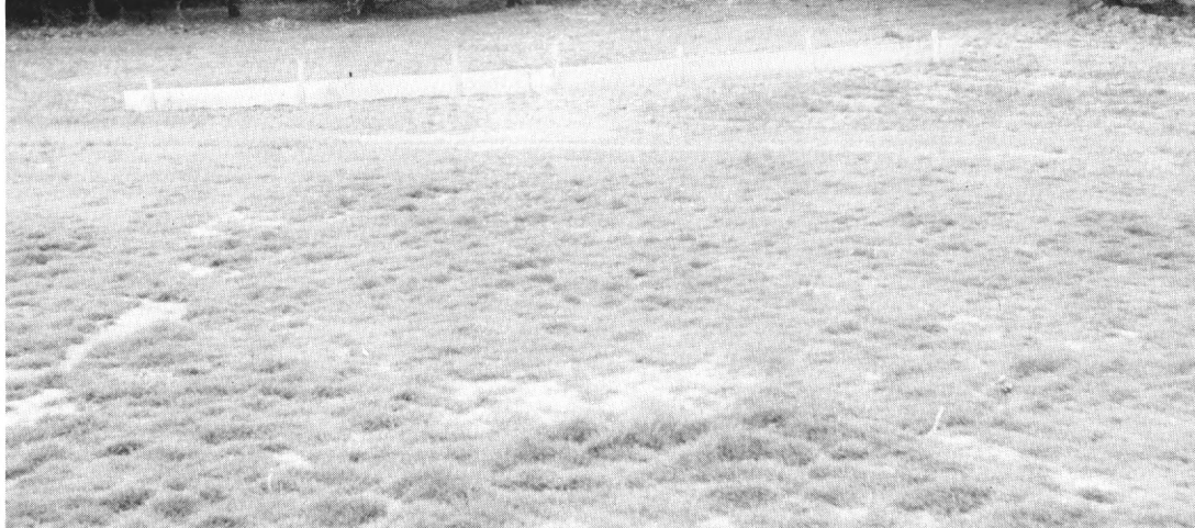
When erosion started during construction, the area was not regraded; boards were placed to divert water. What happens when boards are eventually removed?
