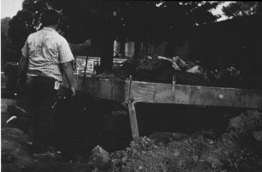
Concrete retaining wall being faced off with rail- road ties.
