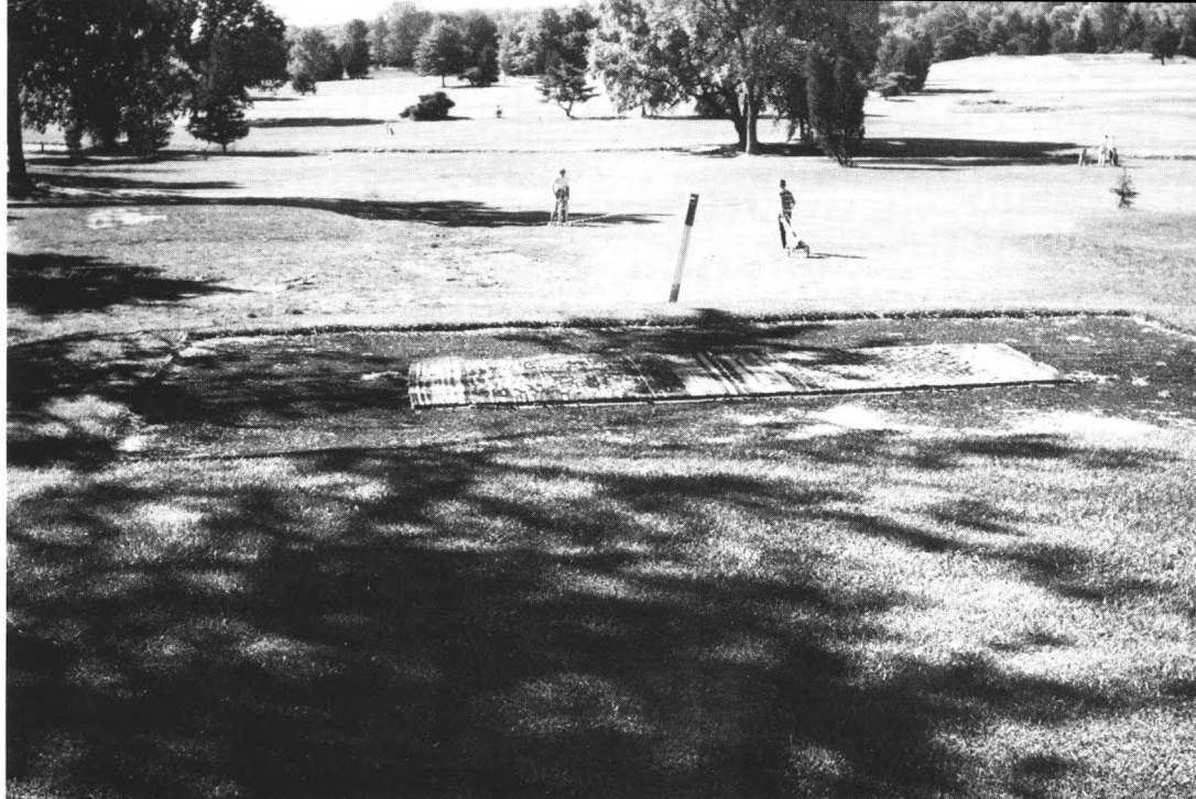
The front portion of this tee is asphalt with rubber mat.
