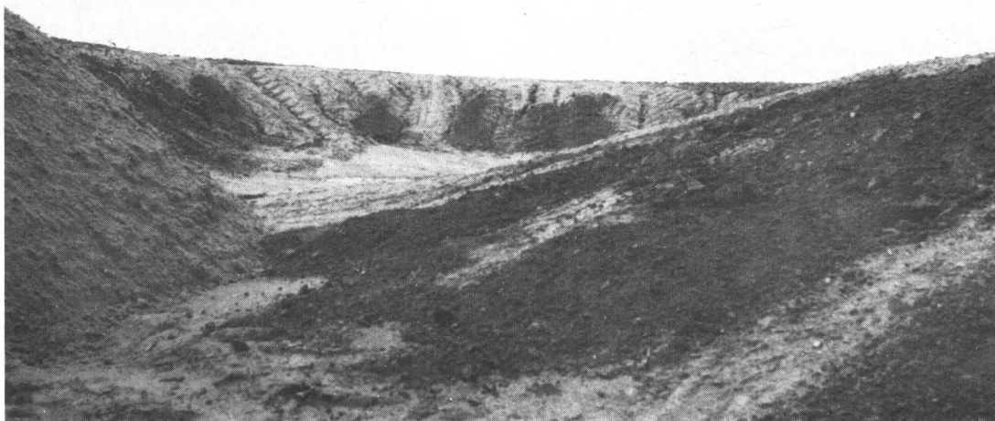
New bunker—very steep construction to hold sand or to mow grass.
