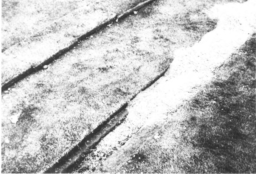
Coarse sand tops off the trench.
