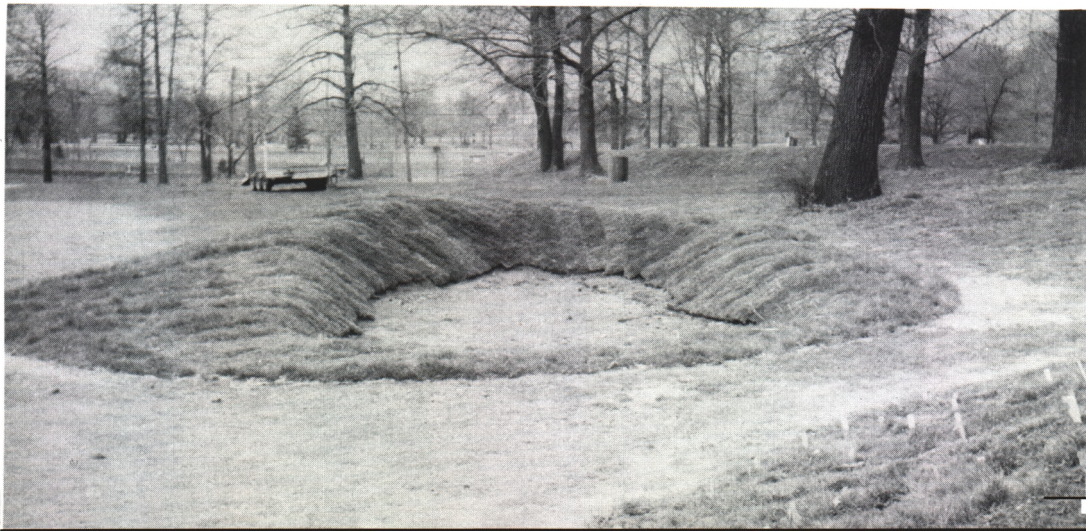
Figure 1. Old style sand bunkers under construction.
