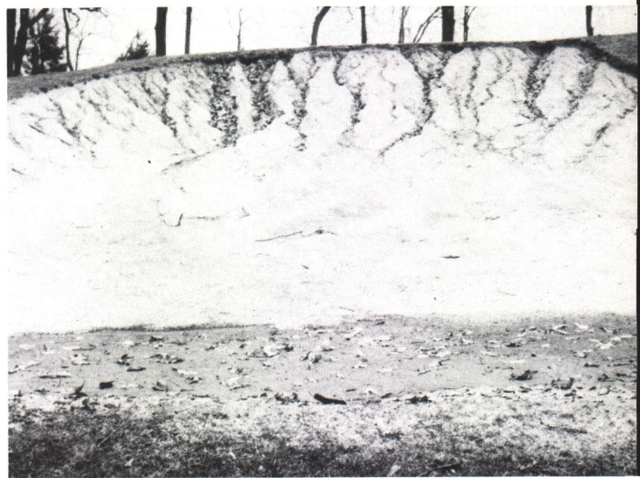
Figure 4. New design sand bunker, with soil erosion problems.
