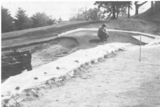
Ringing the green with plastic as an interface between native soil and new greens soil.
