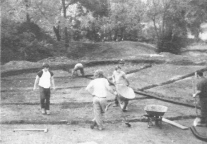
Installing drain lines in the sub-grade.
