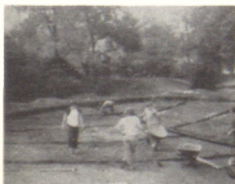
COVER PHOTO—Installing drain lines in the sub grade of a putting green.
