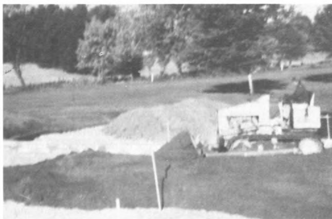
Top soil spreading operation.
