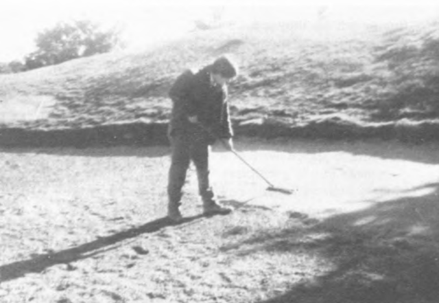
Coarse sand layer being installed over the stone base continues to be an integral part of the construction procedure.
