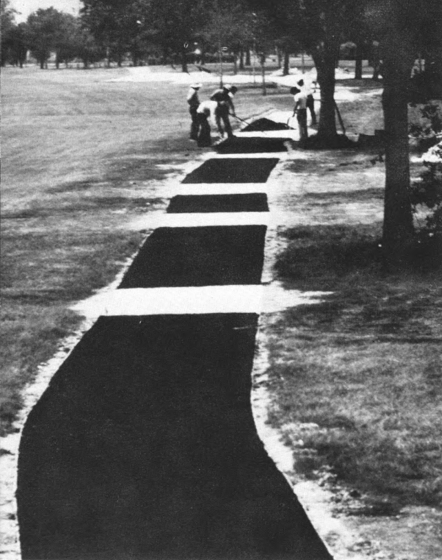
John Biddy at Lakeside Country Club, Houston, Texas, placed concrete in low drainage areas for minimum repair.
