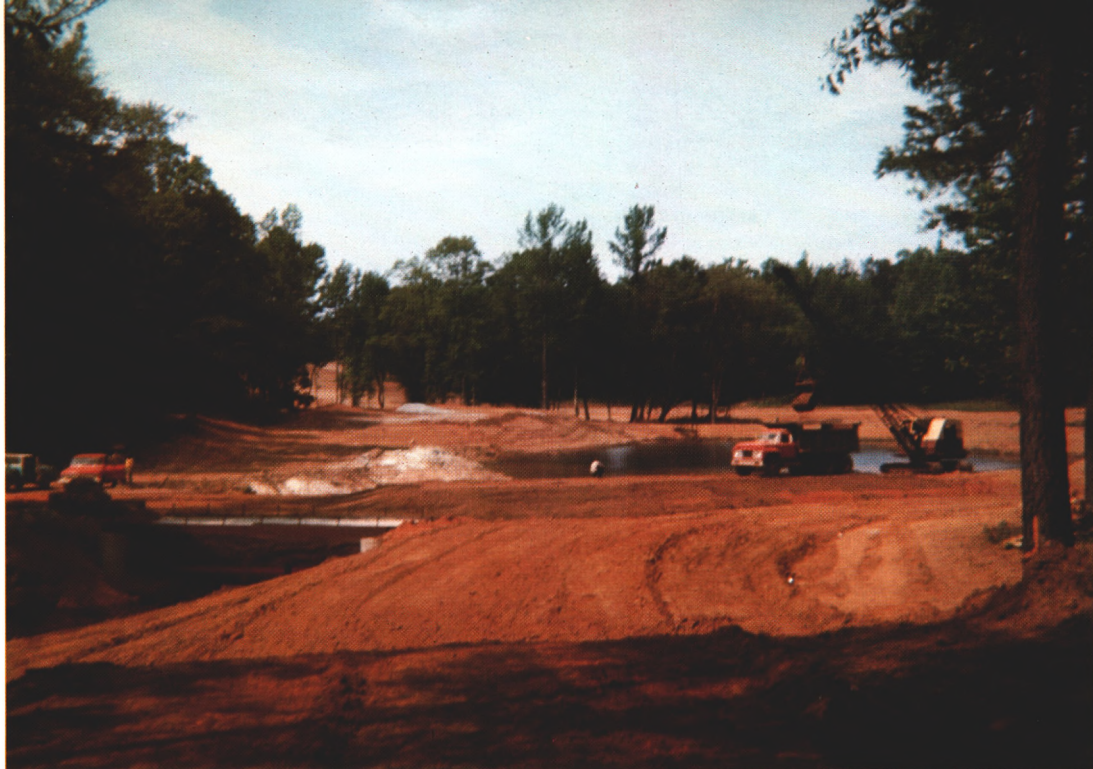
Reservoirs of adequate water-holding capacity are best developed during construction stage of course development.
