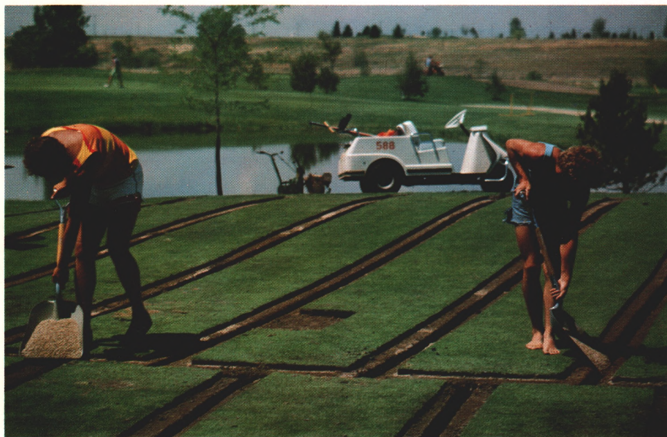
(Top, left) Lateral drain trenching and clean-up.
