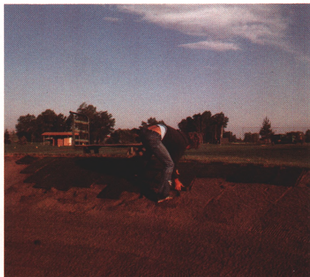
(Below) Preserving the stripped sod by placing it on sand in greenside bunker.
