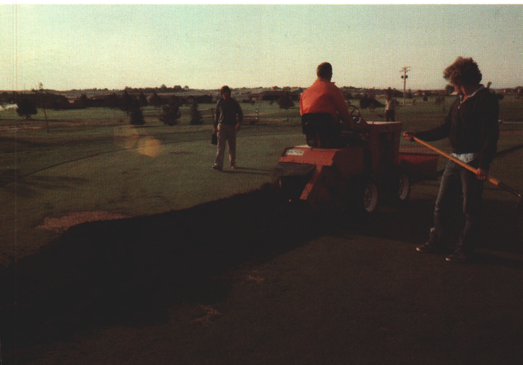
(Left) Trenching for the main line.
