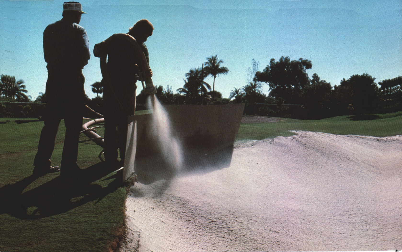
The gunite method compacts the sand in place. The plywood board keeps sand within the bunker.
