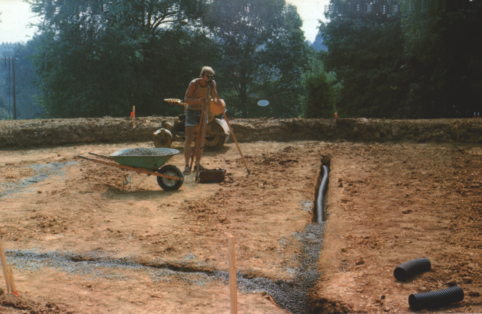
Perforated plastic 4-inch tubing serves as drain line. Worker covers drain with gravel.
