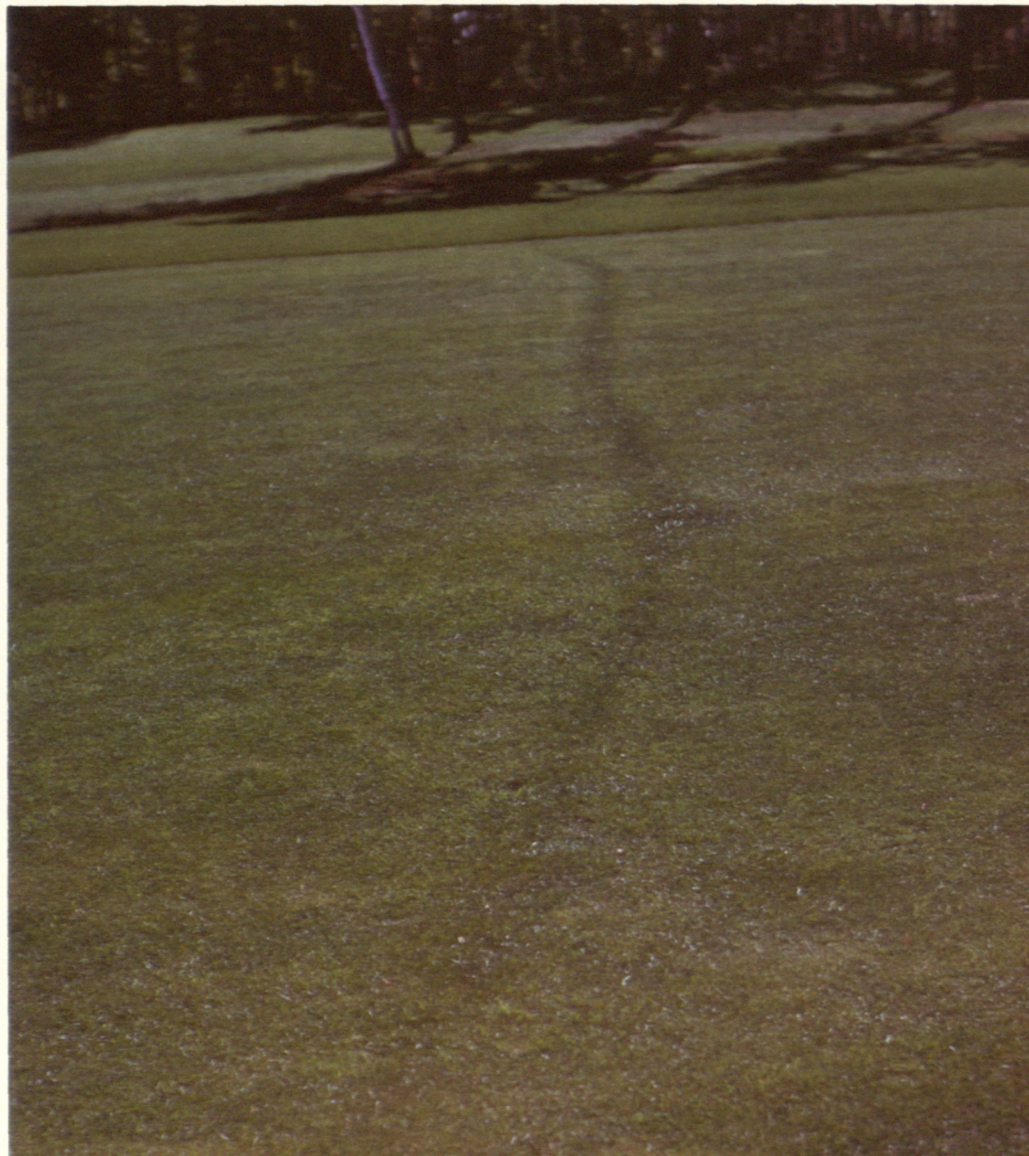
Figure 3. Turf eventually grows over the stone, but this does not impair the effectiveness of the drainage system. Twin Hills Country Club, Massachusetts.
