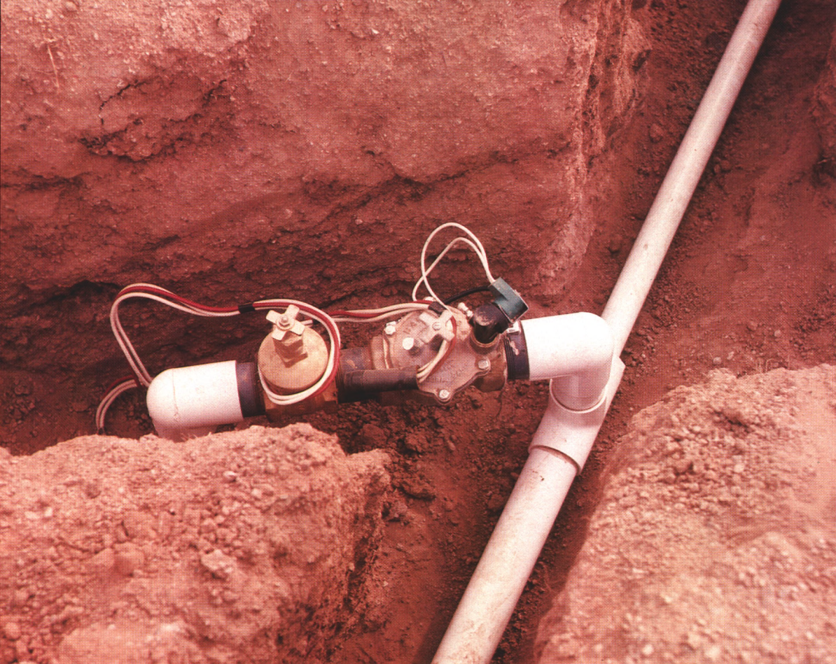
Gate valve and electric valve serving three fairway heads — note slack wire for easier repair of electric valve. Gate valve permits electric valve to be worked on while the system is pressurized.
