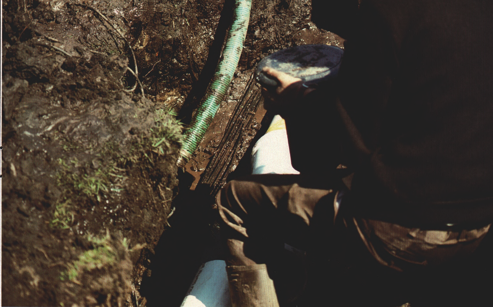
Bundled control tubing makes for easy repair.
