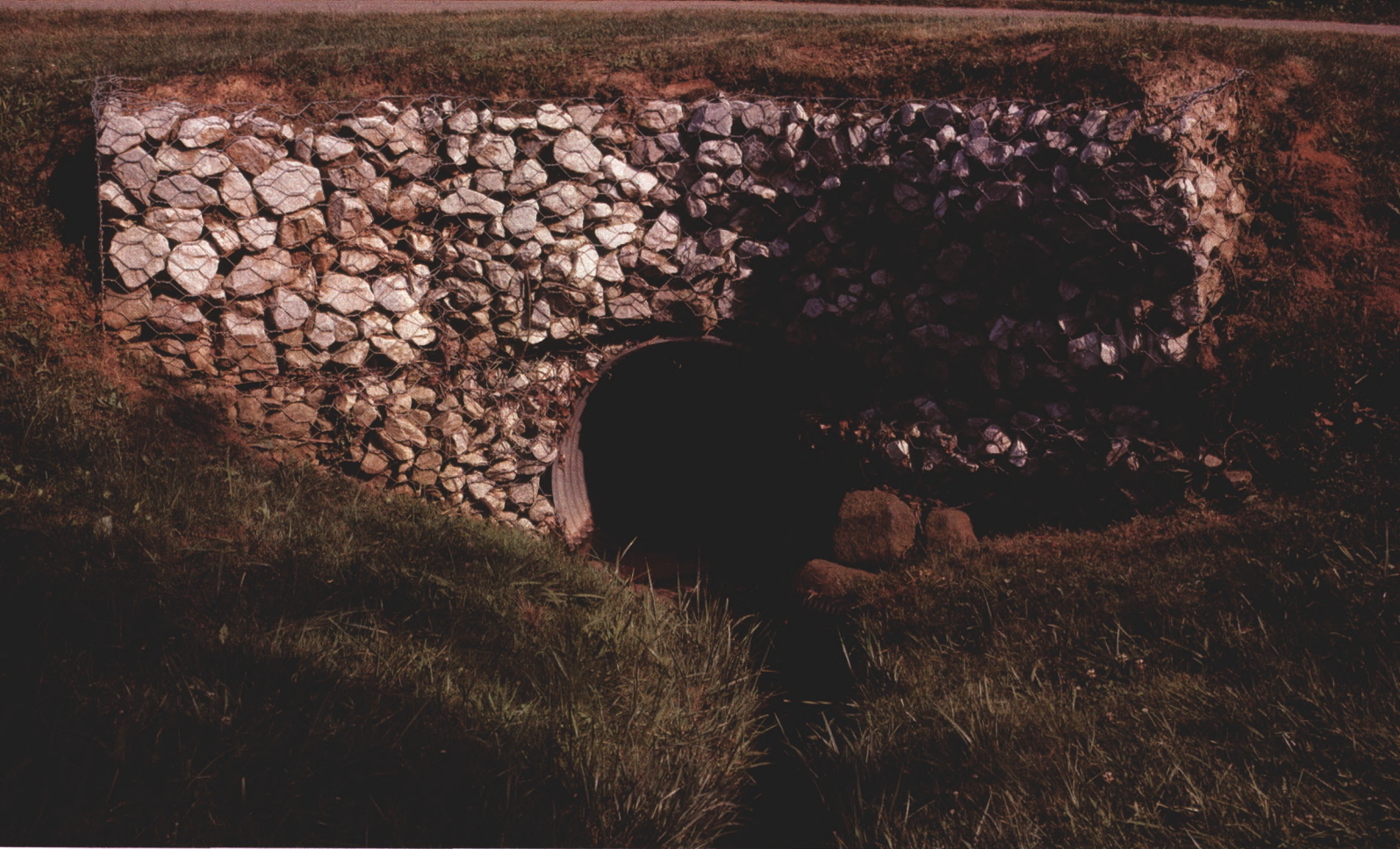
Gabions being used as a headwall.
