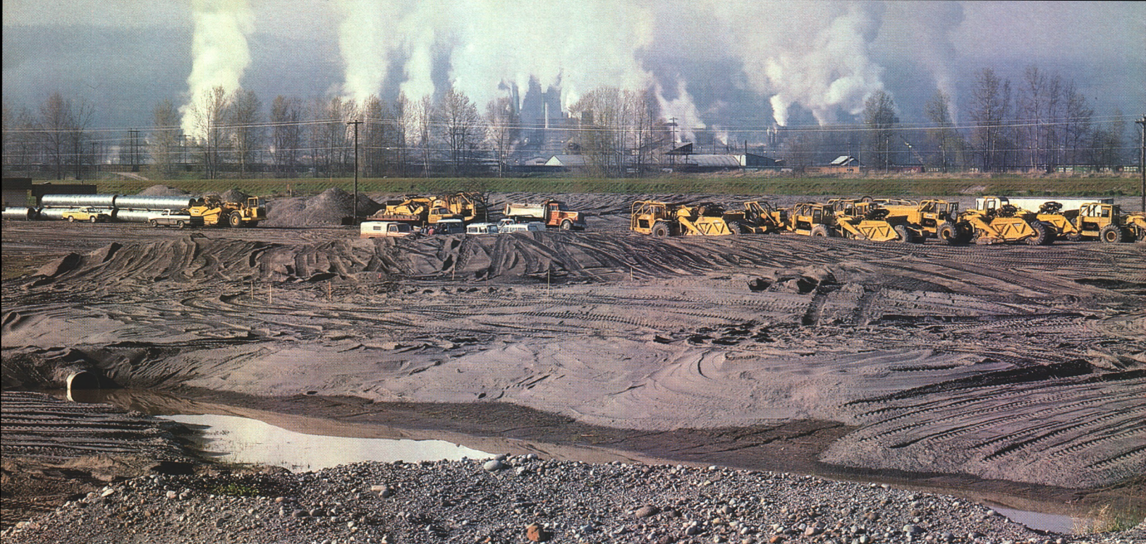
Some of the earth-moving equipment and haul-road culvert used during rough grading for the Kelso course.
