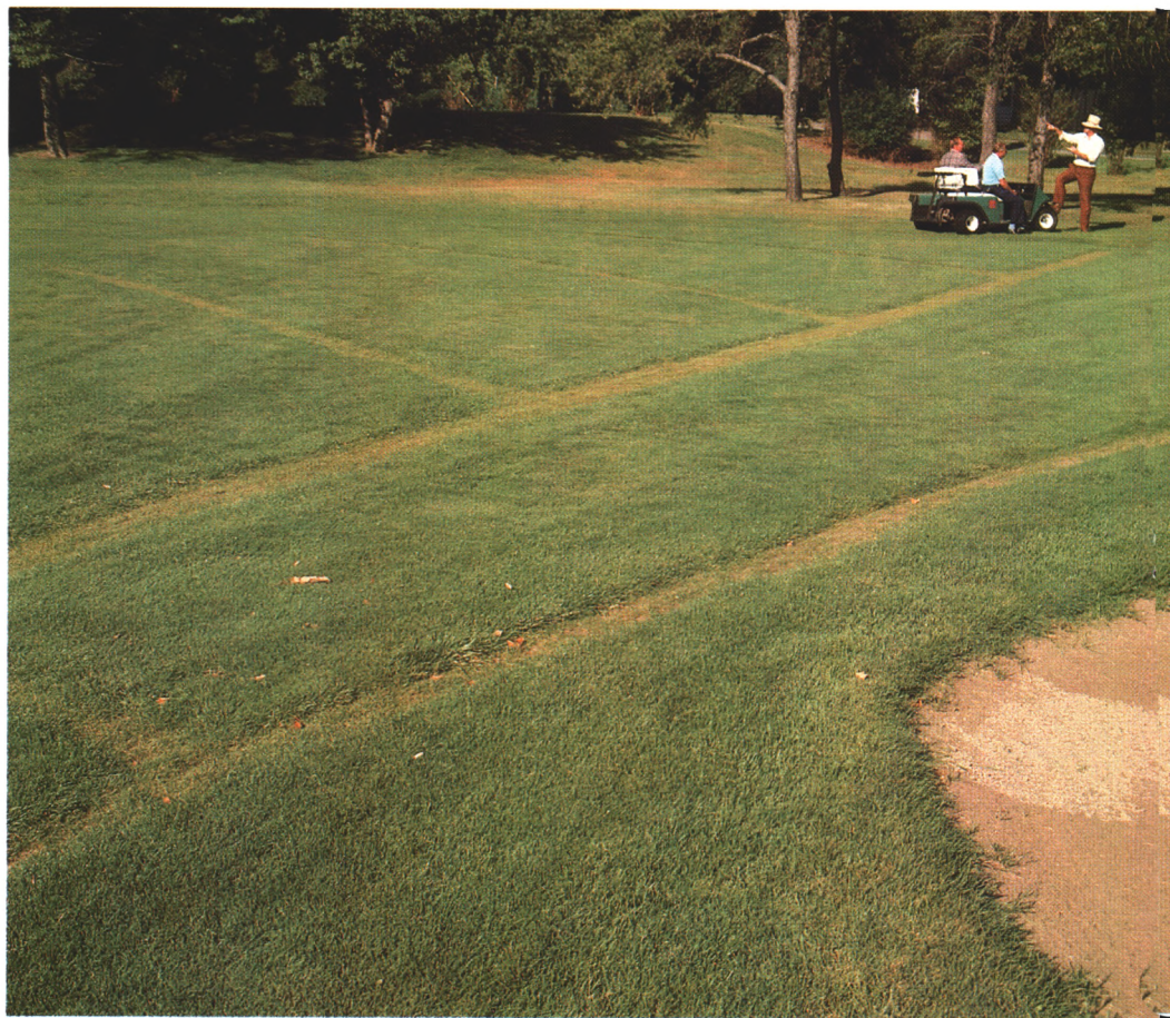
Good drainage is a prerequisite for good turf. Tile and stone-filled trenches are topped off with coarse sand and then seeded at Cherry Hills Club, Ontario, Canada.
