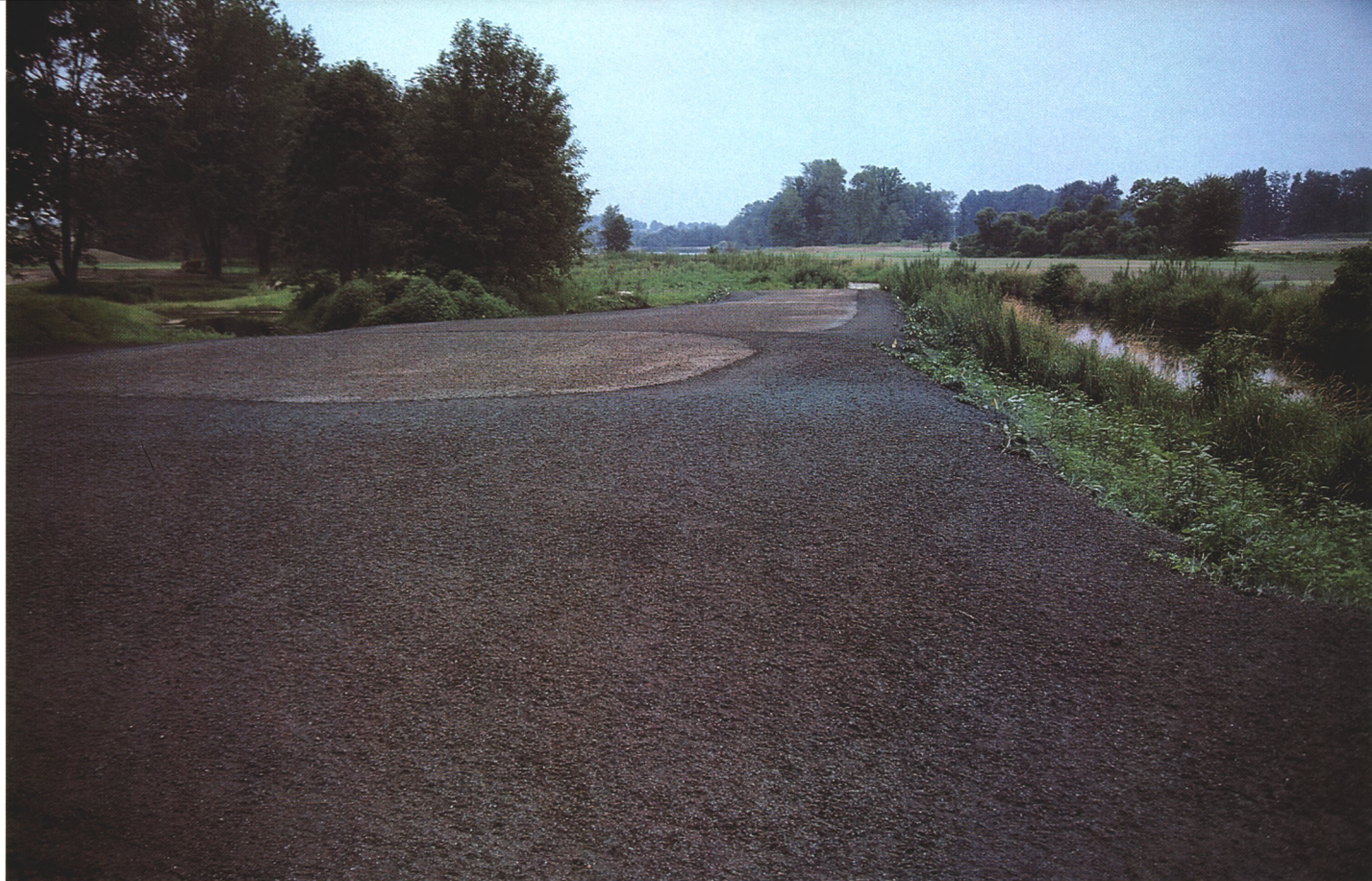
The finished job.
