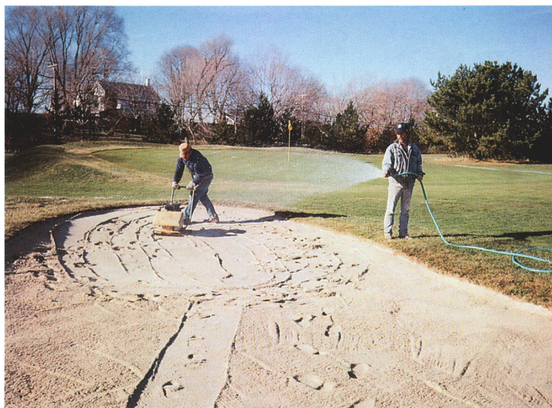
The application of water to the newly installed sand produces an ideal base on which the cement finisher can move.
