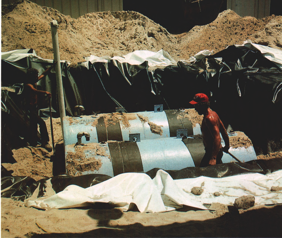
(Top left) Protecting groundwater supplies by installing new fuel tanks with liners and monitoring wells.
