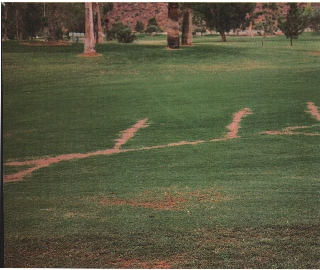
Basic subsurface drainage tile installation is still the most important means of removing excess moisture.
