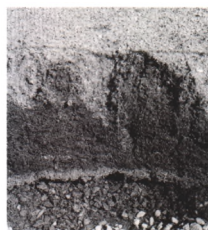
Cover Photo: Profile of a green built to USGA Specs.
