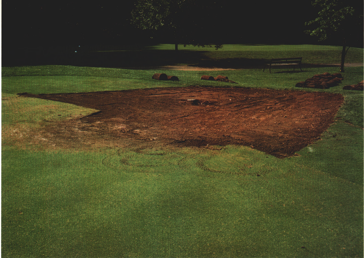
In this instance, poor surface drainage was corrected by removing the sod, regrading the soil, and replacing the sod.
