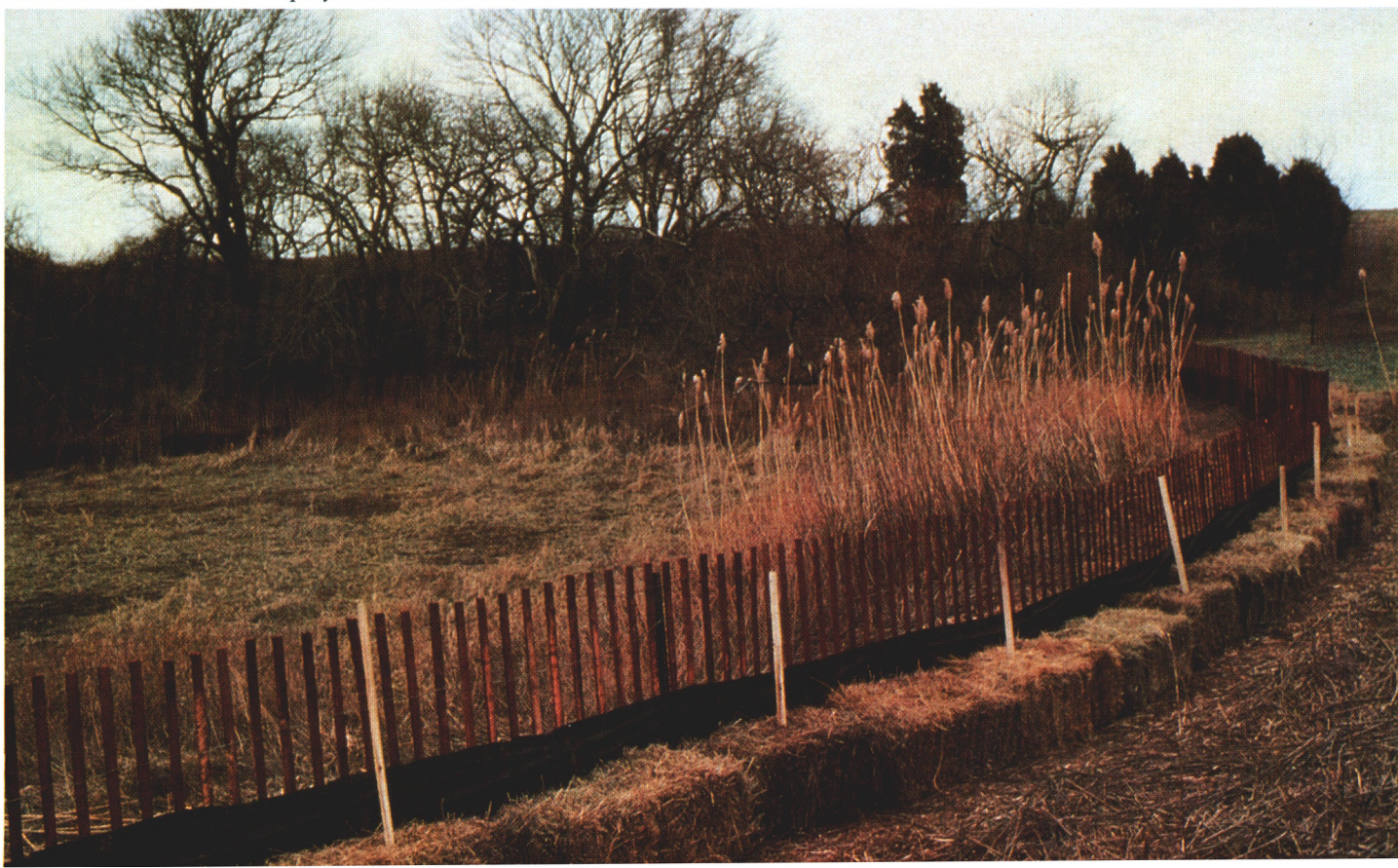
Erosion control methods employed around the wetlands.
