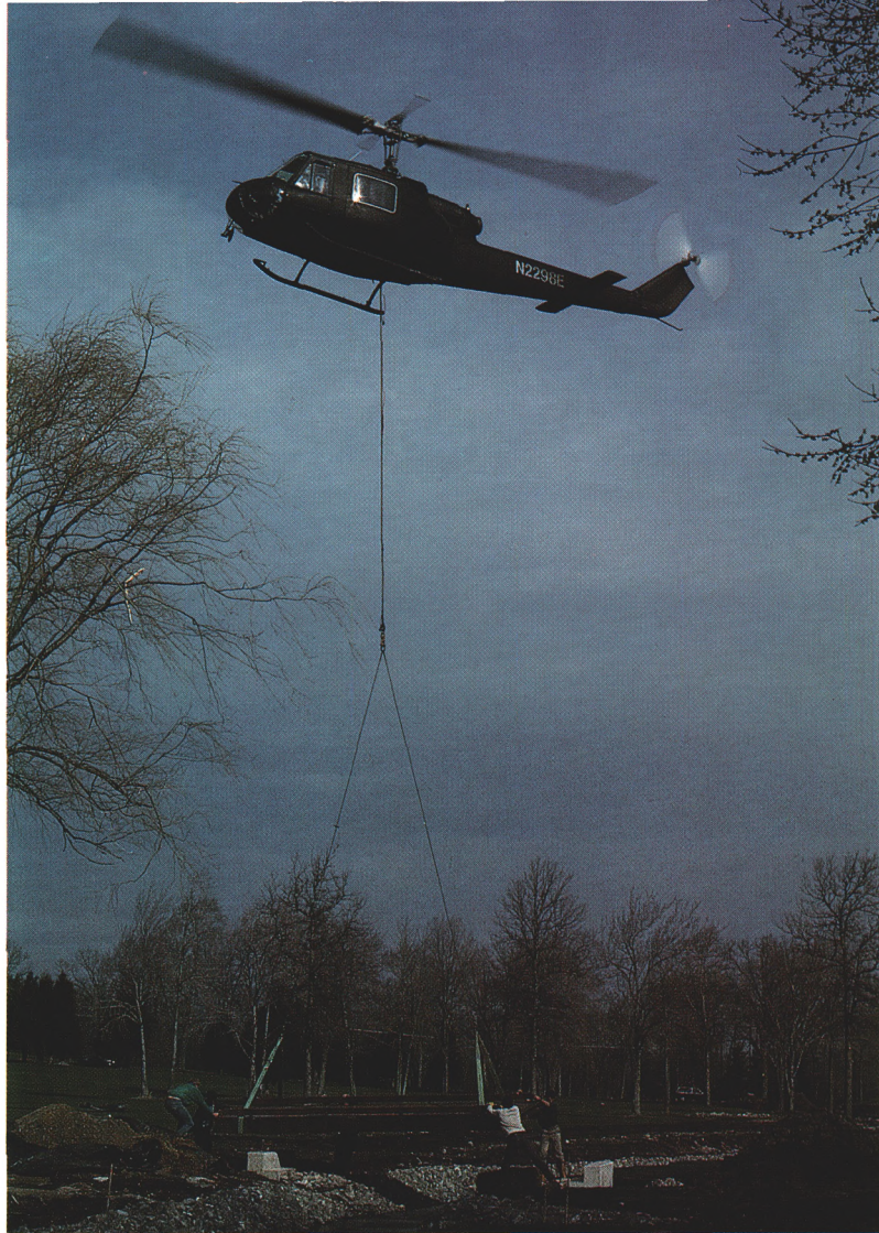
A helicopter effectively moved the bridge when soil conditions were too soft for heavy equipment.
